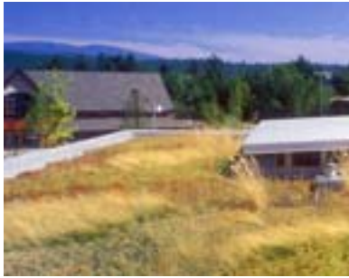
Example of Green Roof
