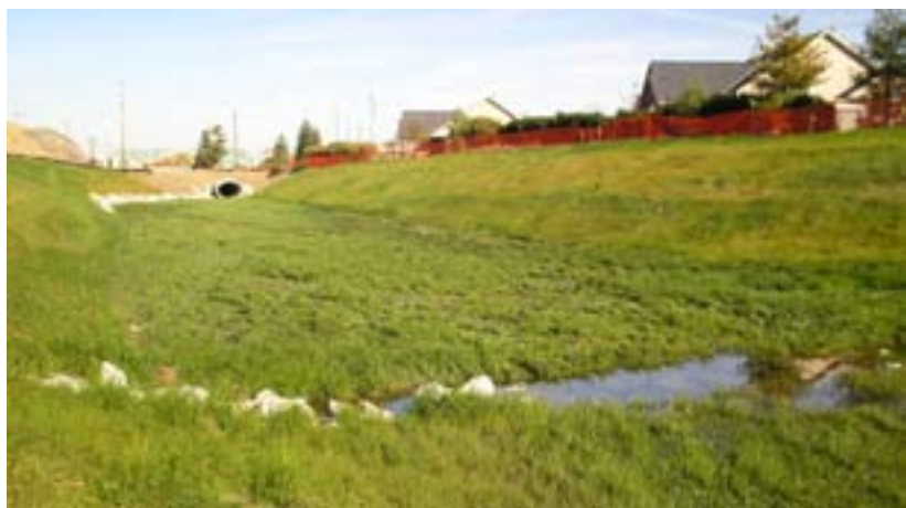
Application of over-wide channel technique.
